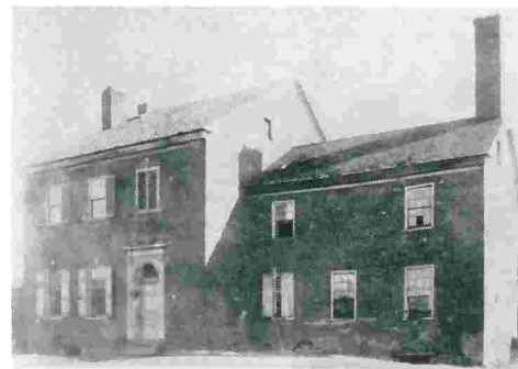
DEER PARK — Built by William Hepburn in 1800, using bricks from his own brick yard.
